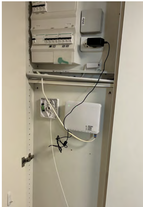
installation i gang
